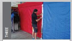
Attach rain gutter strip to marquee wall.
