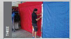
Attach rain gutter strip to marquee wall.
