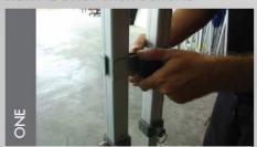
Position marquees side by side and attach leg connector and tighten.
