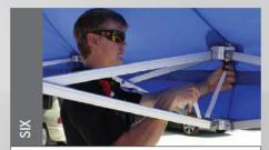
Attach roof straps by looping straps around frame and engaging clip.
