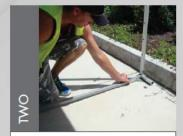
Insert the steel lock bar into the lock connector. Repeat on all four sides.
