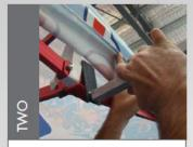
Attach centre support pole to the truss bar of the marquee.
