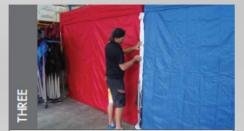
Attach rain gutter strip to marquee wall.
