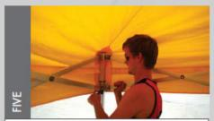
Pull all roof connector pins.
