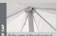
Fit the center of the roof on top of the center pole. If your marquee has a cap pull strings until tight.
