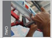
Attach centre support pole to the truss bar of the marquee.
