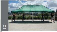
Lift all six roof connectors until pin locks into position.
