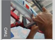
Attach centre support pole to the truss bar of the marquee.
