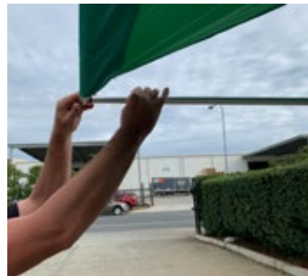
6. Insert the awning poles into the 'holes' in the (three piece) awning pole in sleeve.
