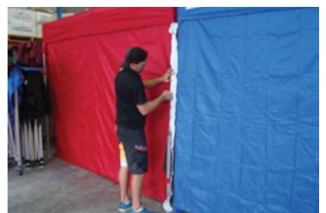
Attach rain gutter strip to marquee wall.
