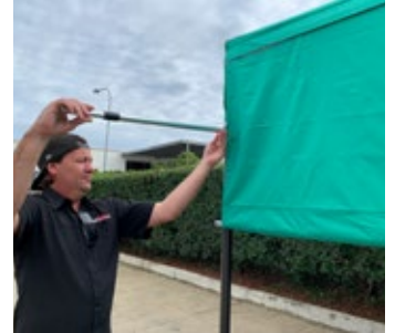
4. Fit the awning end poles to the connector and attached fabric. Repeat on other side.
