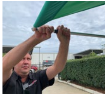
7. Twist the awning poles to extend or shorten and then twist poles to tighten.
