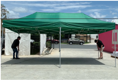
13. Stand on the foot plate and extend back corner legs to desired height. Repeat for middle leg. REFER TO SECURING YOUR MARQUEE.
