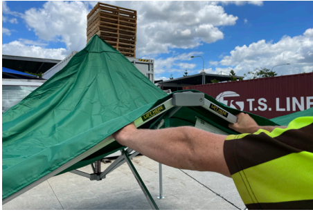
6. Grasp marquee truss bars and walk marquee inwards.
