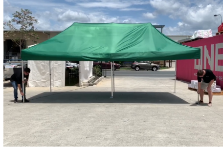
2. Repeat step 1 for the back middle then back corner legs until all 6 legs are lowered.
