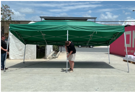
12. Extend the front middle leg to desired height.
