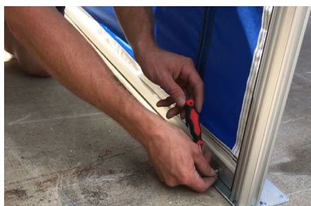
10. Insert Bar connection into the tracking on frame. Adjust the Bar as need to be level and in desired position, tighten bolts to secure. Repeat.
