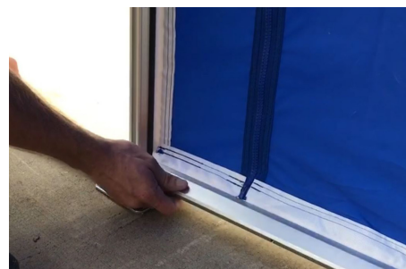
9. Bottom of Full Wall. Insert the Full Wall Keda into the Support Bar and slide Bar along fabric.
