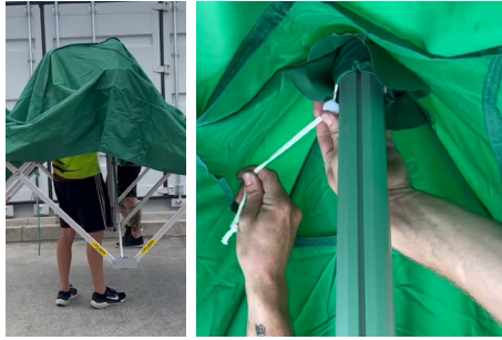
7. Release velcro from the marquee roof from frame. Release roof cap from centre pole and remove roof for transportation.
