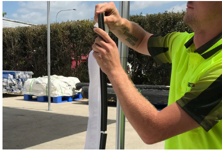
2. Slide the Leg Rubber Inserts (2) along the Keda of the of the Wall Strips. Align to the bottom of Wall Strip.
