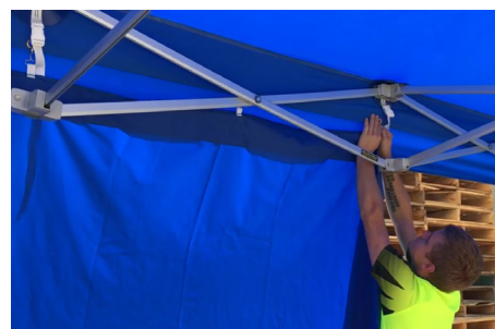
6. Full Wall Panel attach the Hooks to the Eyelets on Roof. Ensure Hook is facing inwards.
