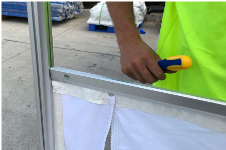
7. Insert the Wall Strip Keda into the Half Wall Bar. Insert the Half Wall Support Bar into the Tracking of the Upper Leg of the Canopy.
