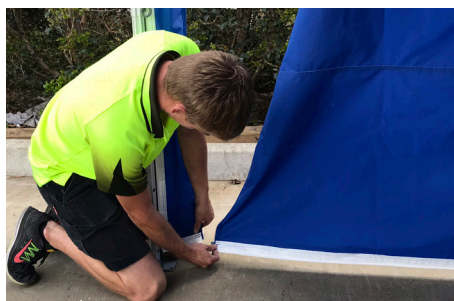
7. Zip the Wall Strip and the Half Wall Panel together. Repeat on other side.
