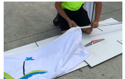
6. Top of Half Wall. Insert the Half Wall Keda into the Half Wall Support Bar and slide fabric along Bar.
