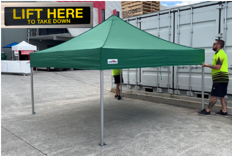
5. Push to release all roof connector pins & Refer to 'LIFT HERE' To Take Down' sticker on the Marquee. CONTINUE TO NEXT PAGE >>
