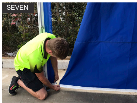
SEVEN Zip the Wall Strip and the Half Wall Panel together. Repeat on other side.
