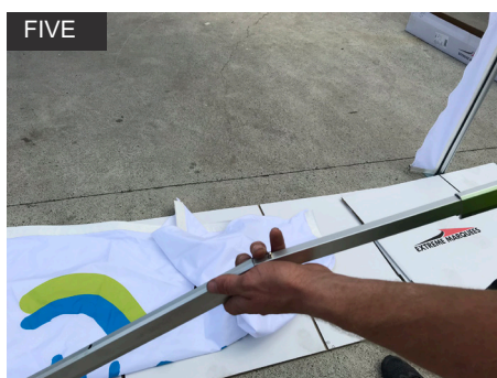
FIVE Assemble the Half Wall Support Bars for the top and bottom of the Half Wall.
