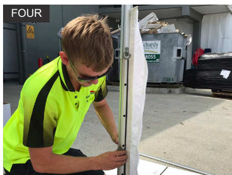
FOUR Press the Leg Rubber Inserts into the tracking on the Lower Leg of the Marquee. Repeat on other side.
