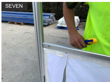
SEVEN Insert the Wall Strip Keda into the Half Wall Bar. Insert the Half Wall Support Bar into the Tracking of the Upper Leg of the Marquee.
