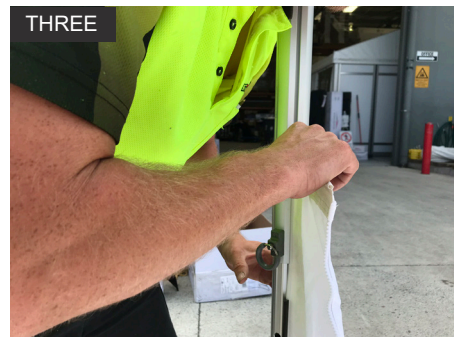
THREE Insert the top section of the of the Wall Strip Keda into the tracking of the Upper Leg of Marquee.
