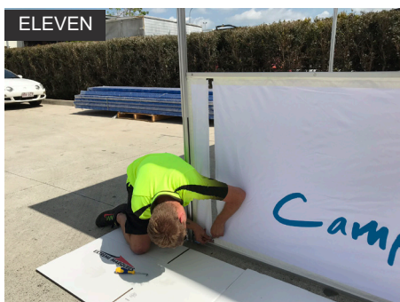
ELEVEN Zip the Wall Strip and the Half Wall Panel together.
