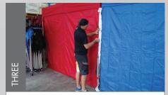
Attach rain gutter strip to marquee wall.
