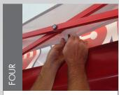
Attach awning clips to inner flap on marquee roof.
