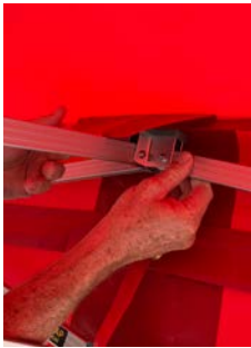
10. Ensure protective flaps are over the truss connectors. Attach them by looping the straps around the truss and engaging the clips, then tighten.
