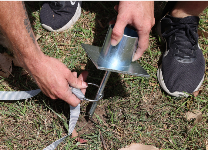
1. Loop one end loop of the stringline through the foot plate spike.
