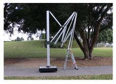
3. Using a step ladder place roof fabric over the Cantilever frame.
